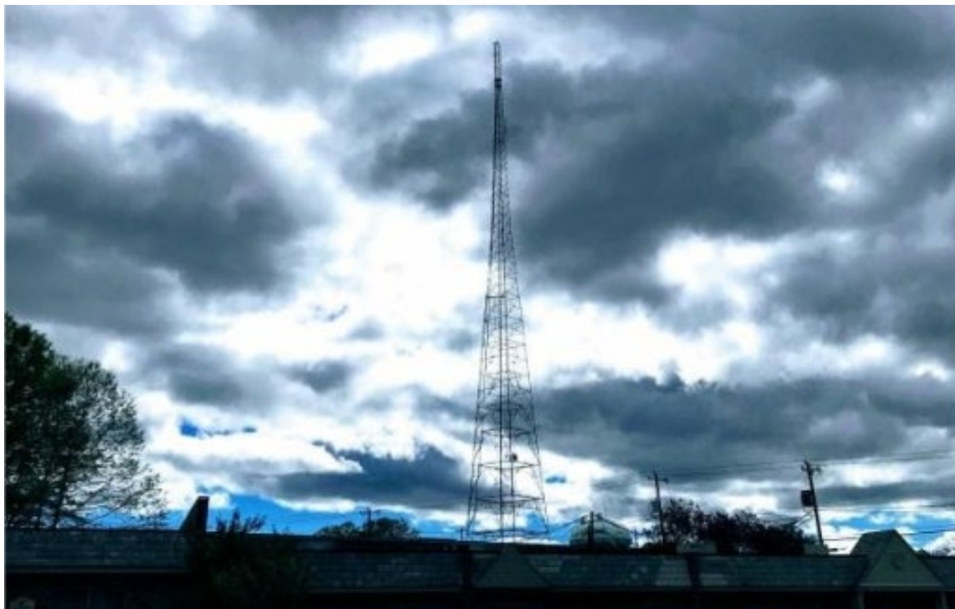
WHKY AM antenna tower
