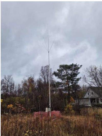
**Comrod antenna for 1314 kHz East of Transmitter House at LKB LLE.**
